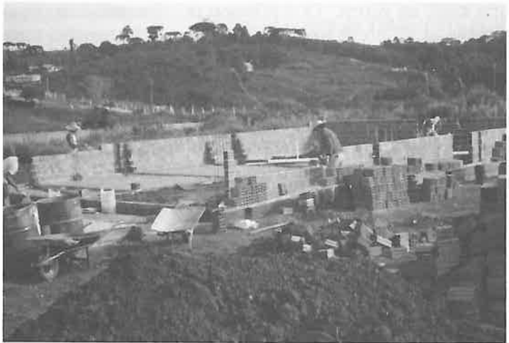
Pastor Teo's house under construction.
